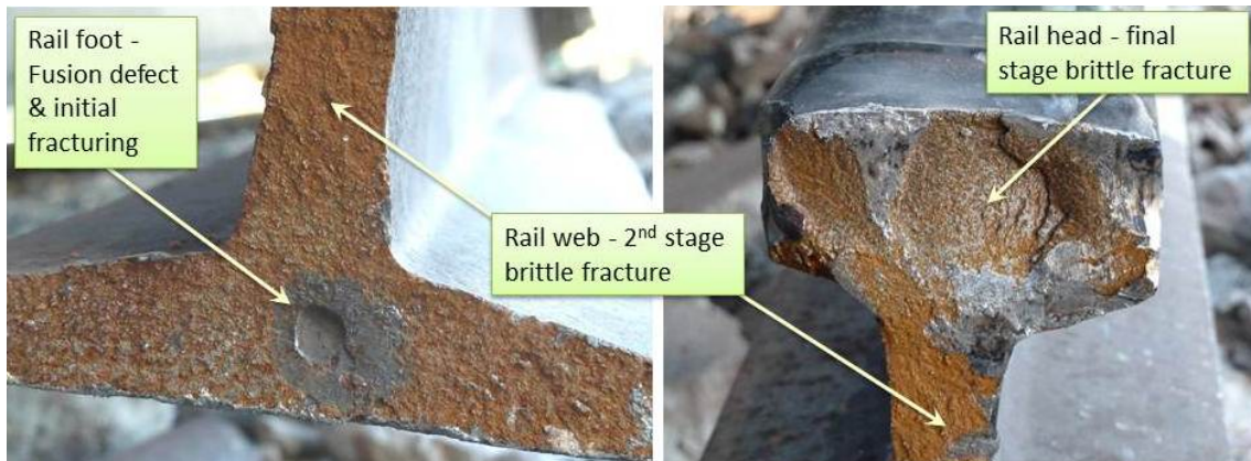
Figure 4: Flash-butt weld fusion defect and brittle fractures
